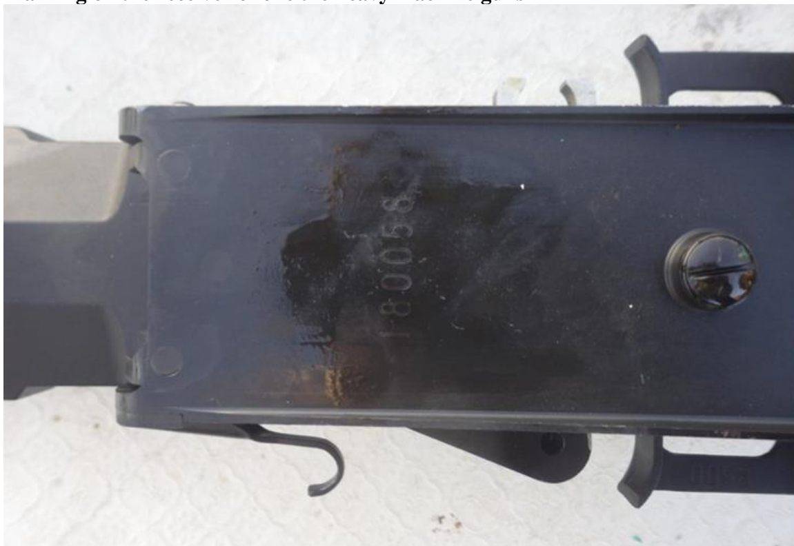
Figure 19.13 Marking on the receiver of one the heavy machine guns
